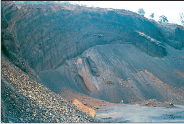
Figure 42. Quarry in an andesitic scoria cone in the footwall of the Pastores fault in the southern part of the map area (see Figs. 3 and 40). Quarry cut is ~20 m high.
